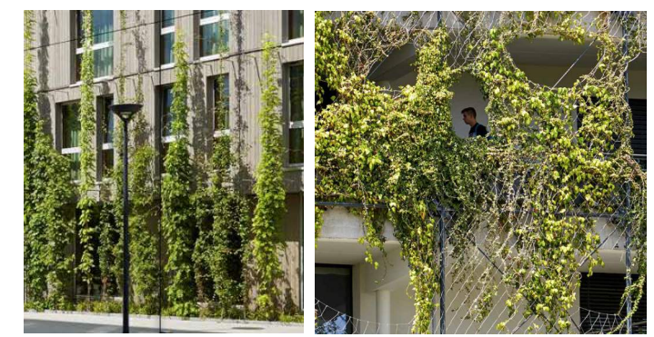
GREEN SCREEN: WIRE ROPE (LEFT), WIRE MESH (RIGHT)
