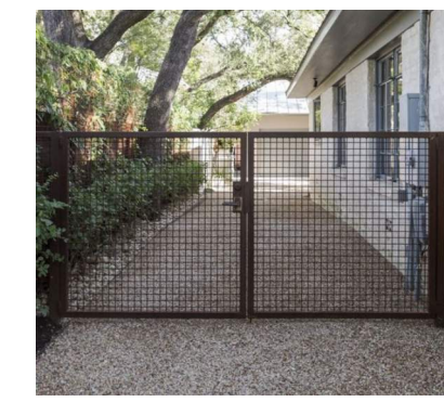
WELDED WIRE MESH FENCE
